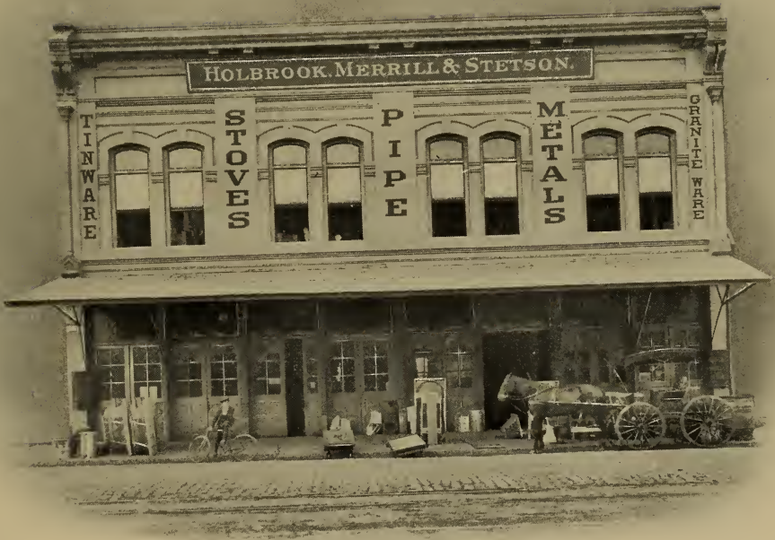
LOS ANGELES HOUSE.
